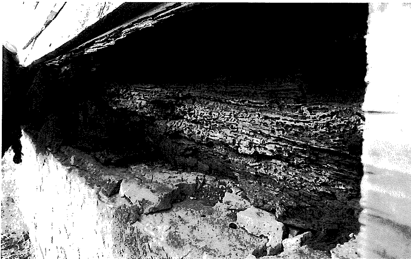
S-1 Deteriorated sill, east side (2017)
