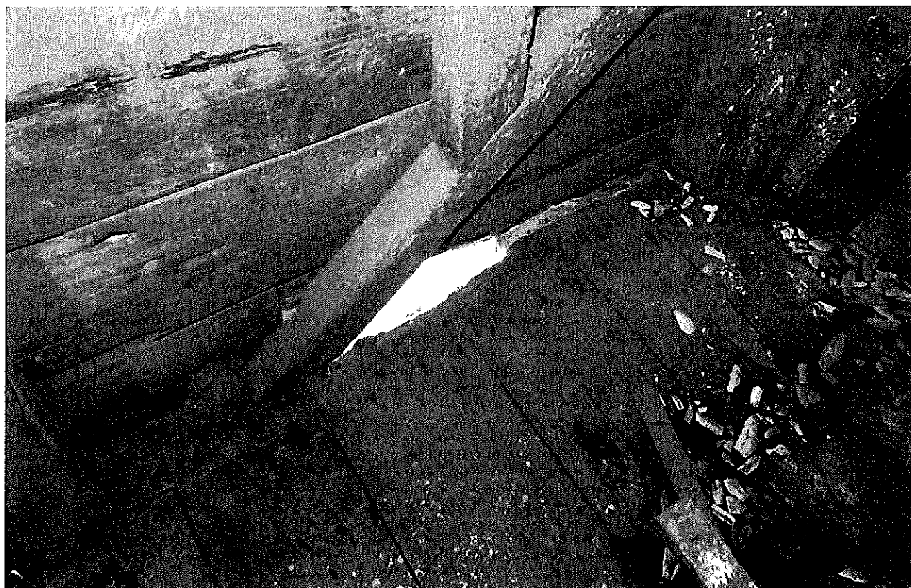
S-1 Deteriorated sill, north-east corner (2017)
