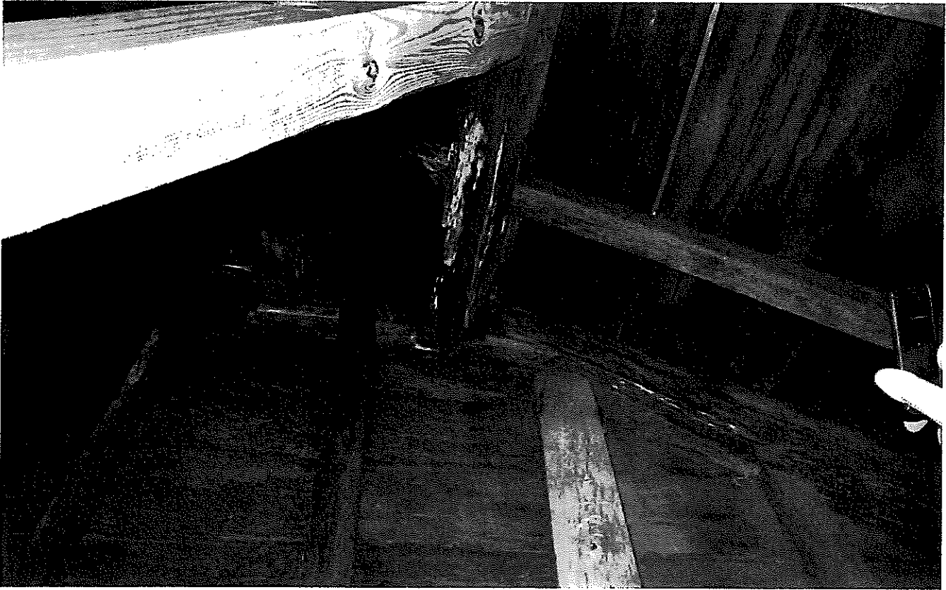
S-3 Deteriorated rafter and purlin connection on east slope of north wall with shoring (2017)
