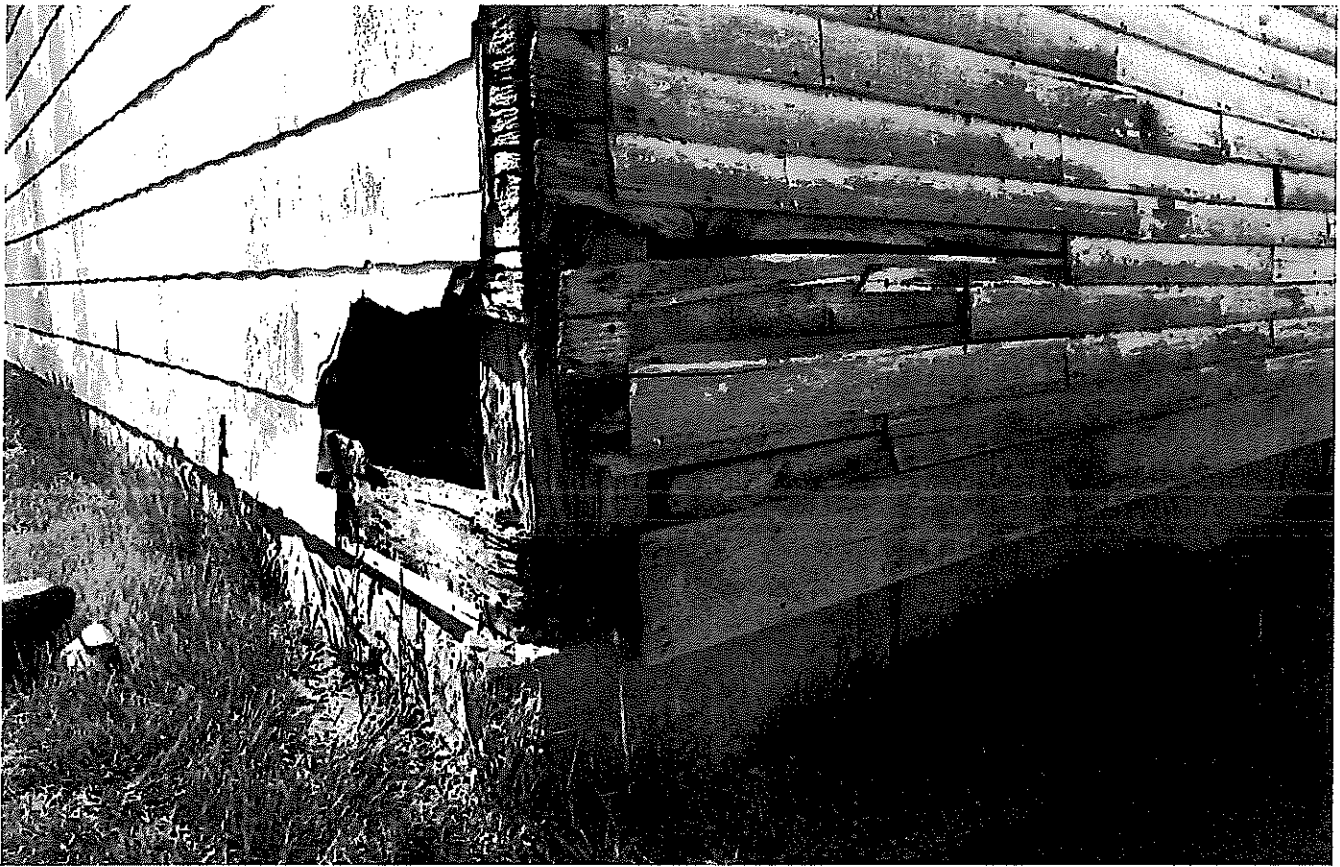
S-2 Deterioration at south-east corner (2017)
