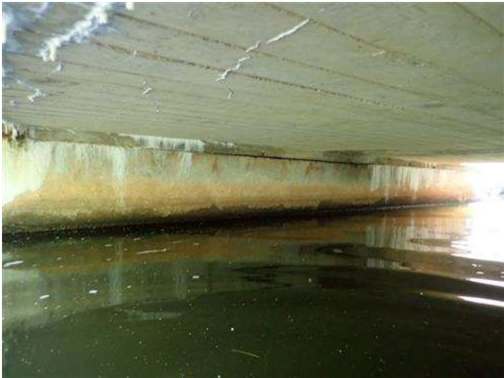
Typical cracking on abutment #1.
