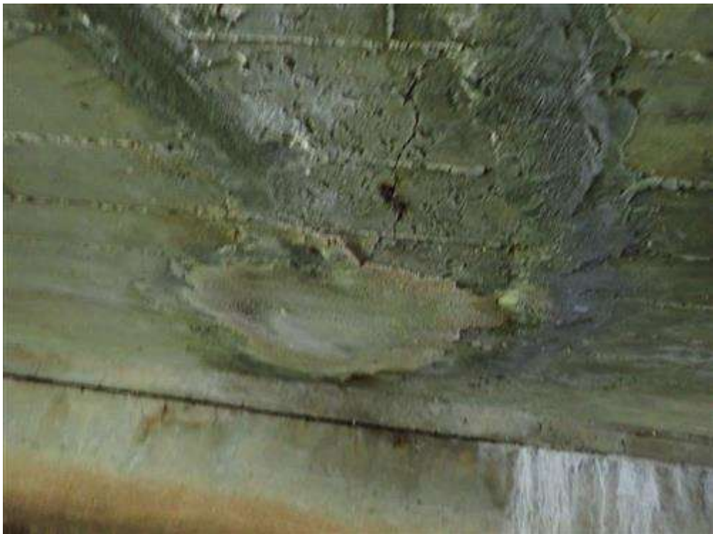
Large patch midspan near A-2 with hollow areas and longitudinal cracks.
