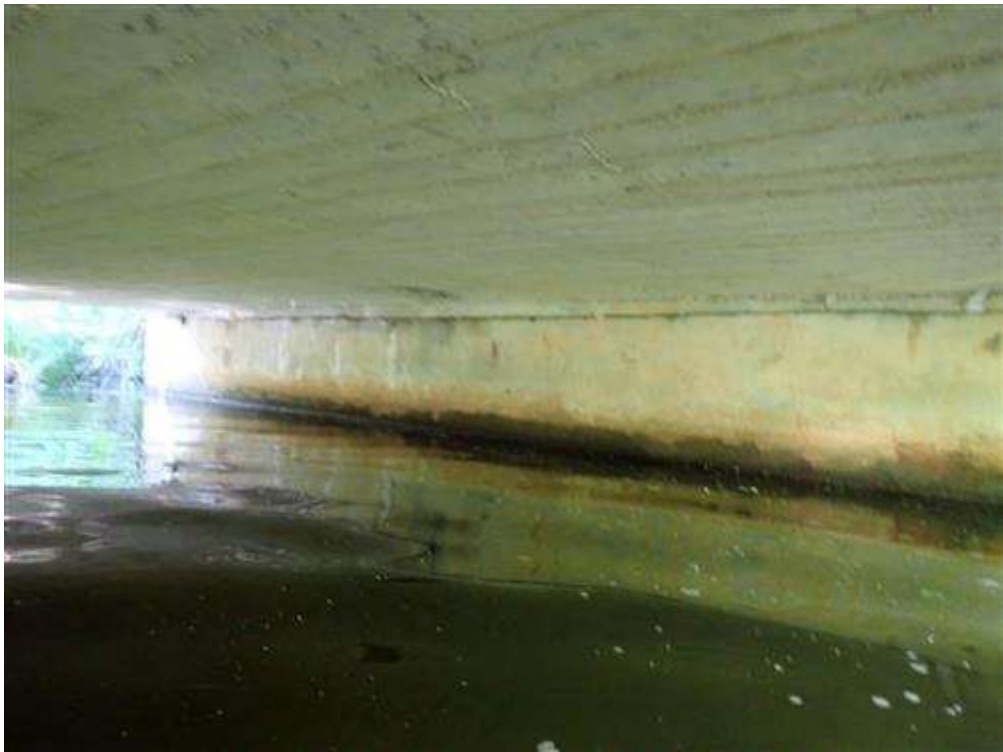
Large patch midspan near A-2 with hollow areas and longitudinal cracks.
