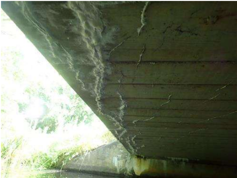
View of cracking on deck underside at the outlet end.
