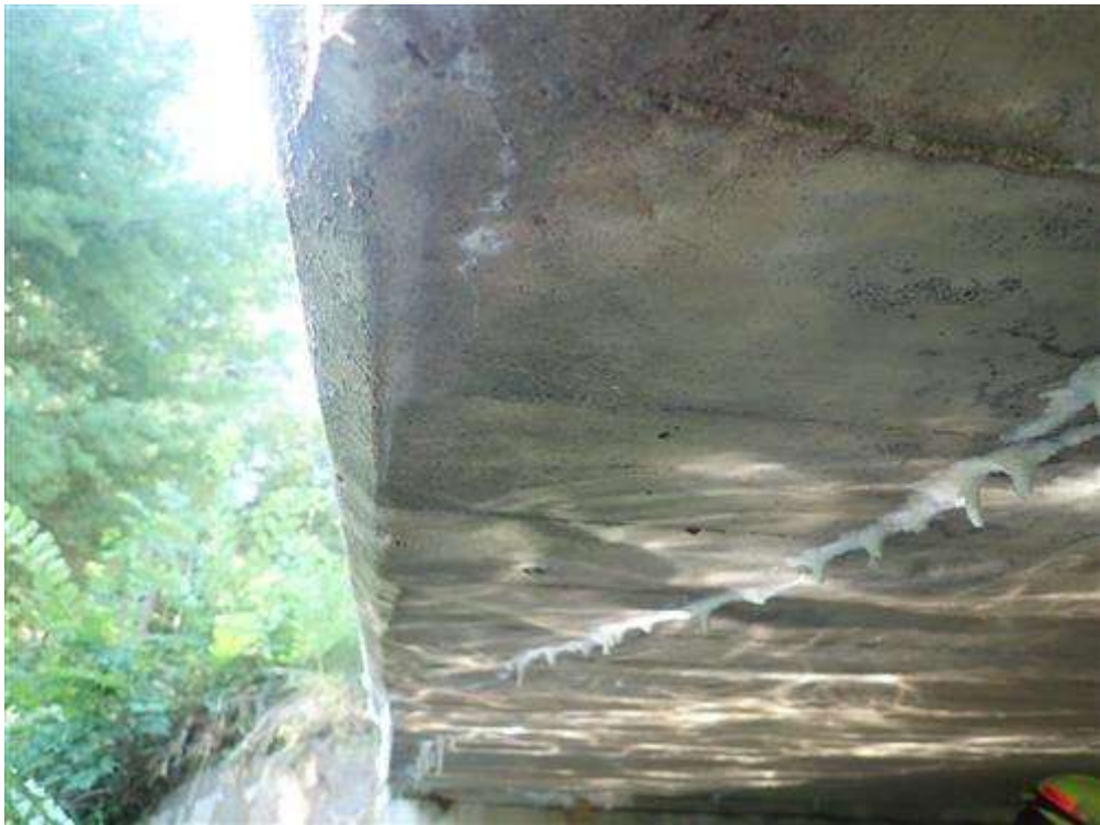
View of cracking on deck underside at the inlet end.
