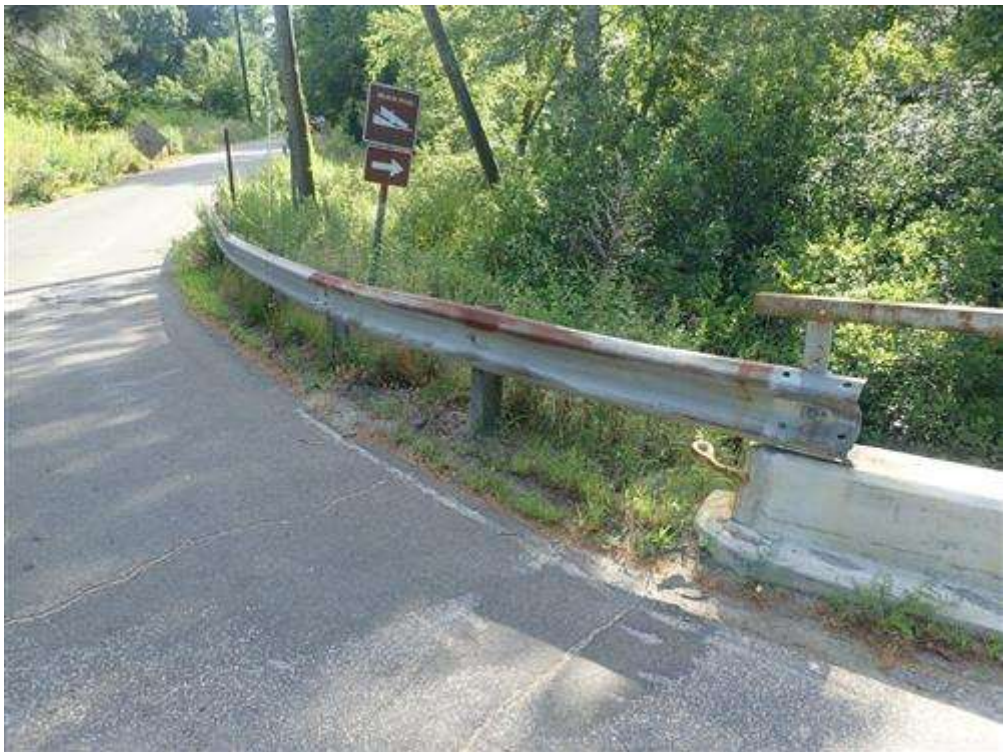
Southbound trailing end approach rail.
