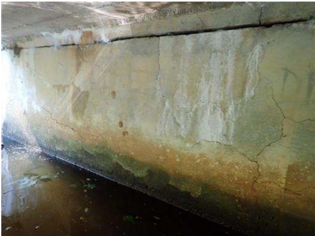
Typical cracking on abutment #1.
