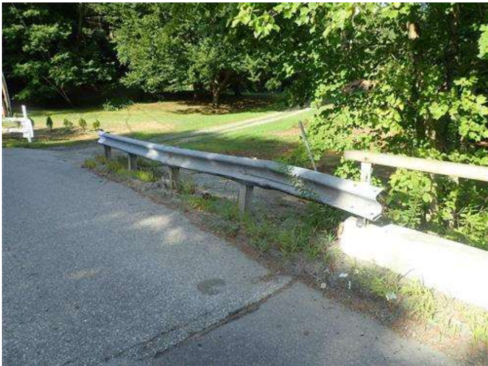
Southbound trailing end approach rail.
