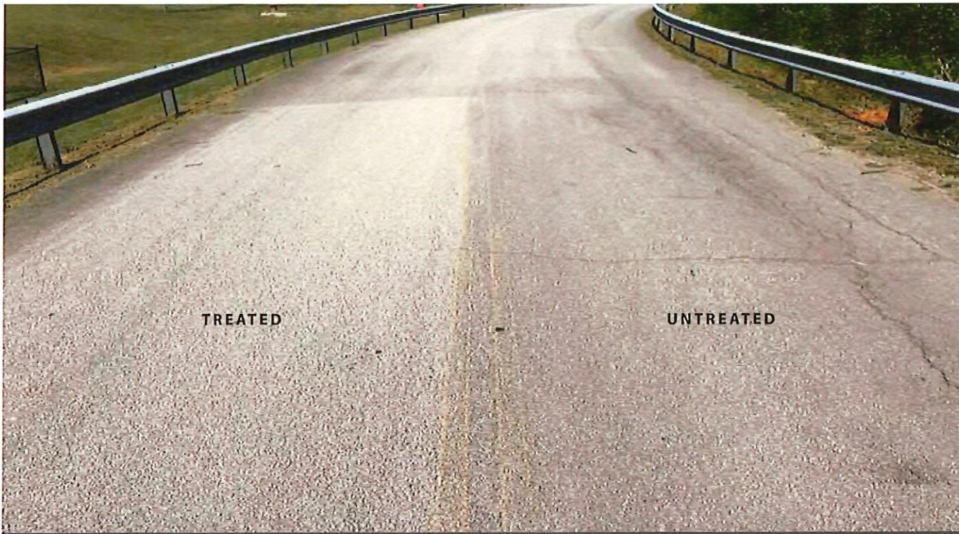
*A section of this roadway was treated with **Reclamite®** in 2003; the balance was not. The photo was taken in September of 2019—16 years later!*
